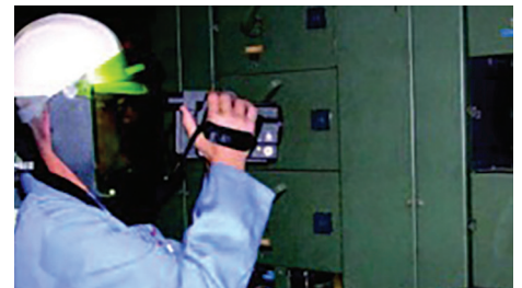
Infrared thermographers look for hot spots that could indicate loose connections and other electrical problems.
